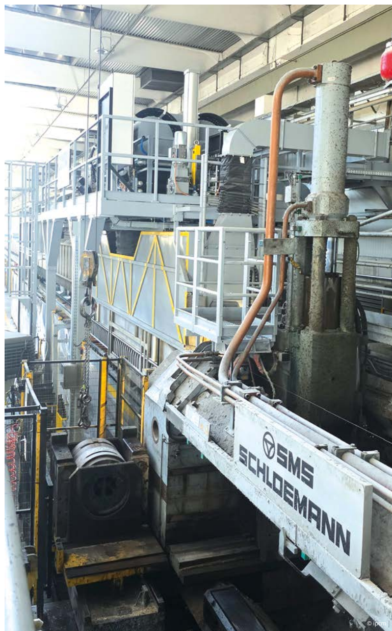
One of the 5 extrusion presses operated by Estral at its Manerbio (Brescia, Italy) site.
