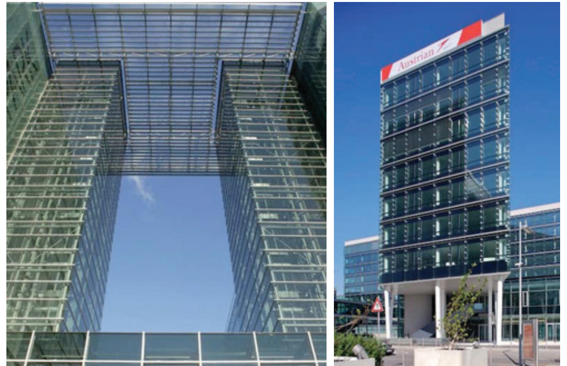
© Photography (2) | Felix Friedmann | GIG Fassaden GmbH
