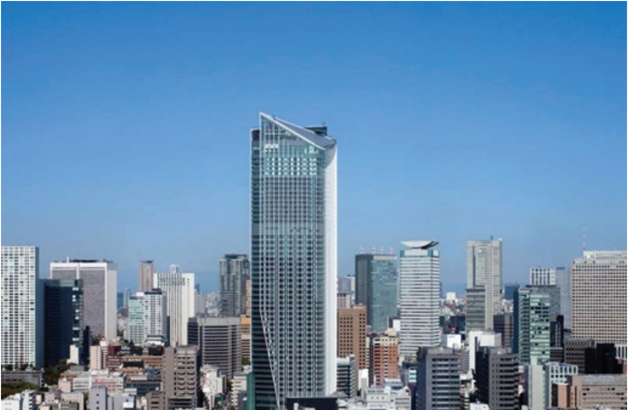
© Photography (2) | Felix Friedmann | GIG Fassaden GmbH
