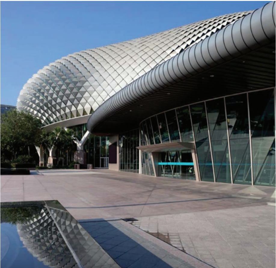
© Photography (2) | Felix Friedmann | GIG Fassaden GmbH
