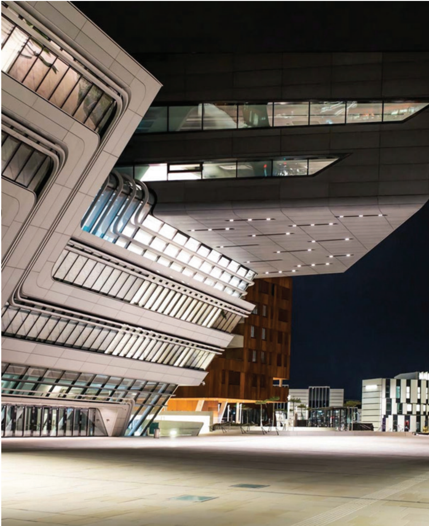
© Photography (2) | Felix Friedmann | GIG Fassaden GmbH
