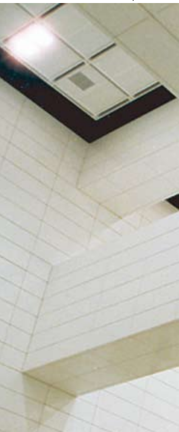
TSING YI STATION, HONG KONG
