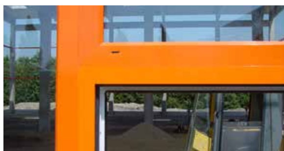
Fig. 4.1.1 Different color due to varying film thickness
