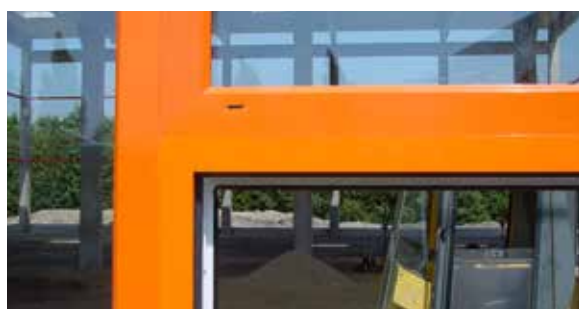
Fig. 4.1.1 Different color due to varying film thickness
