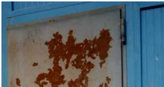
Fig. 5.2.3 Scale, flash rust, white rust
